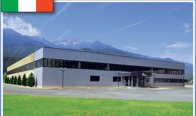
AUTOBLOK manufacturing plant Caprie-Torino
