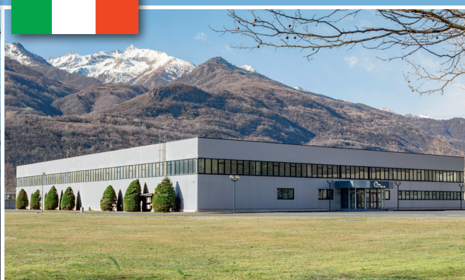
AUTOBLOK manufacturing plant Caprie-Torino
